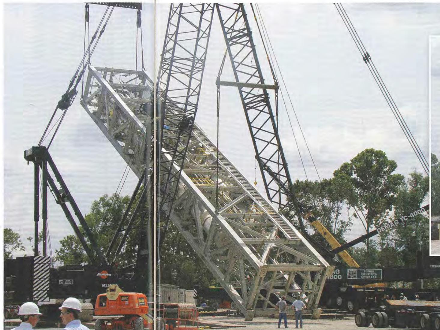
A Manitowoc crawler lifts the largest module upright and places it on the steerable dolly for transport
