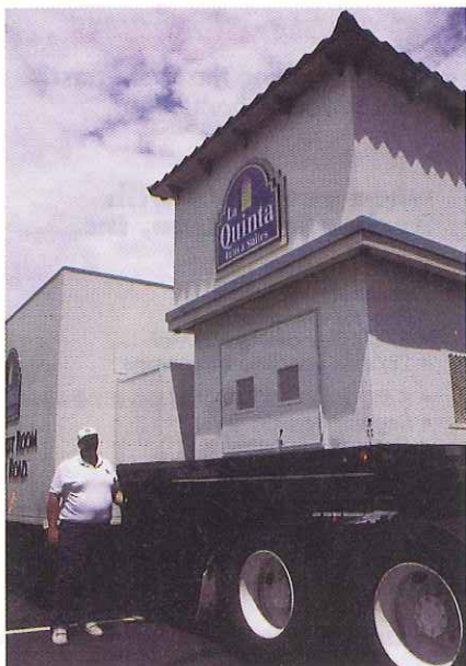
The bell tower on the 30,001st room can be raised and lowered to reach legal height restrictions.
