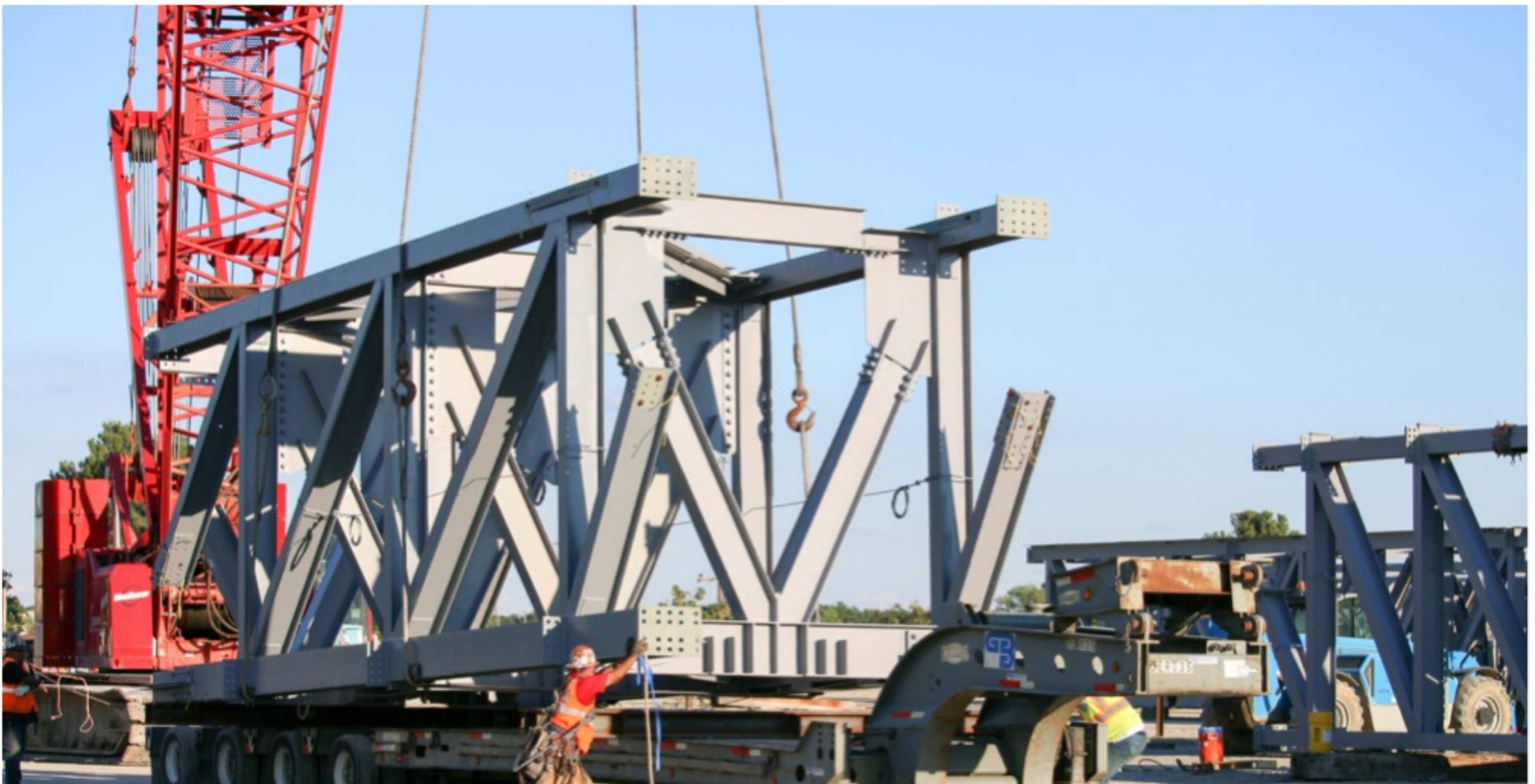
A box truss is lifted onto a flatbed. Hundreds of trusses were welded together to support the roof of the stadium.
