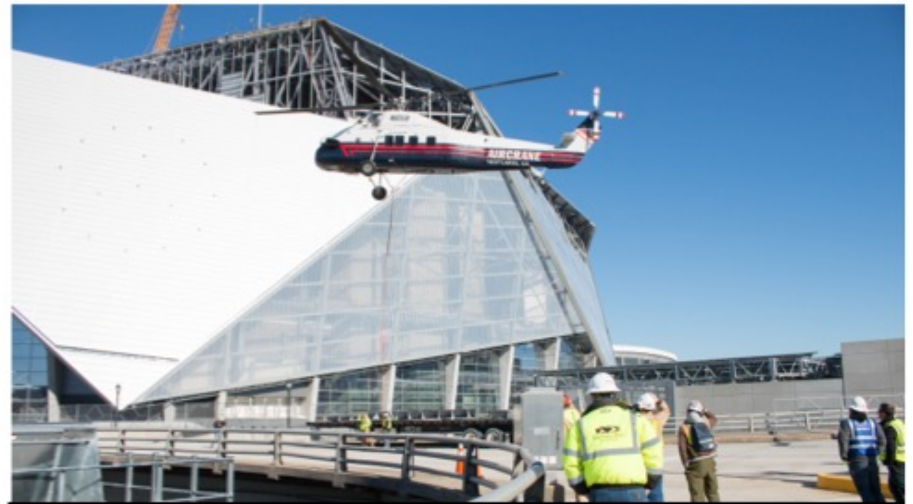
A helicopter lifts a piece of steel off a Bennett flatbed for transport to the roof.
